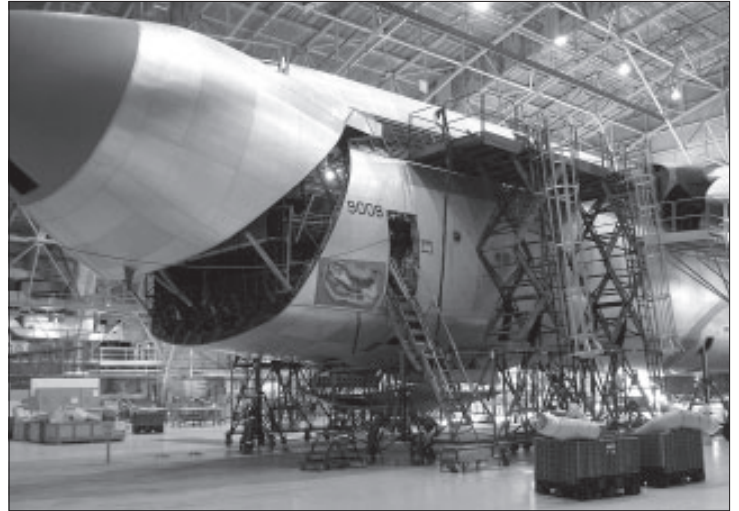
A 105th Airlift Wing C-5, aircraft 9008, undergoes a complete refurbishment and Programmed Depot Maintenance (PDM) in Georgia. The project was completed in six weeks and 105th Maintainers saved the Air Force over $100,000. Courtesy photo.
