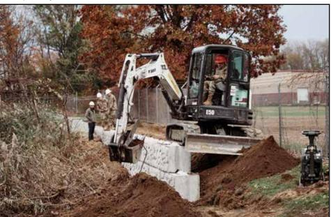
Soldiers assigned to the 1156th Engineer Company headquartered at Camp Smith, N.Y., excavate the foundation for a track built at the New York National Guard headquarters in Latham, N.Y., Nov. 5, 2019. The new track was constructed to give personnel at the facility an option for running that will keep them away from local traffic.
