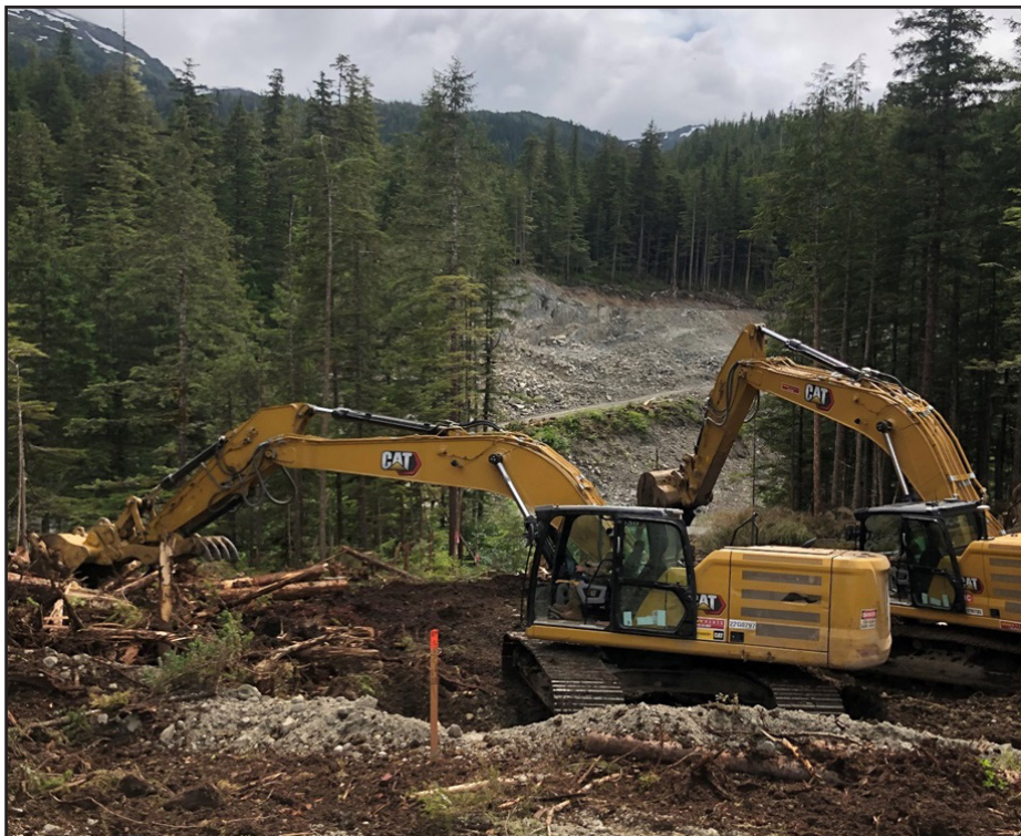
New York Army National Guard Spcs. Logan Storrings and Thomas Butera, members of the 204th Engineer Battalion Quarry Platoon, guide two excavators grubbing out a roadway in rugged terrain near Cordova, Alaska June 20, 2024.
