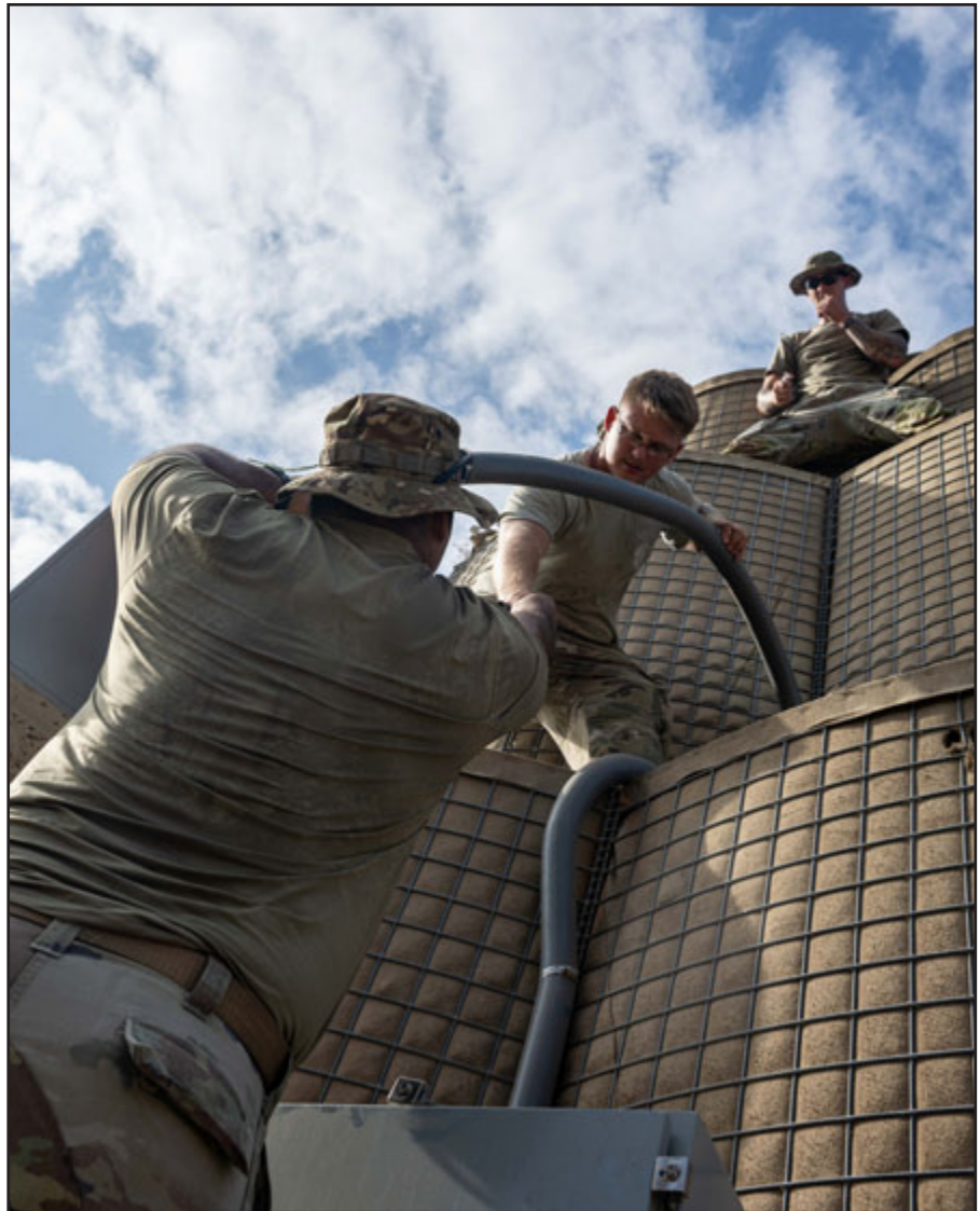
U.S. service members in 152nd Engineer Support Company, assigned to Combined Joint Task Force - Horn of Africa, improve base infrastructure at Manda Bay, Kenya, March 26, 2025. The mission of the 152 ESC is to enhance regional stability and strengthen relationships with partner nations through various construction projects coordinated across East Africa.
