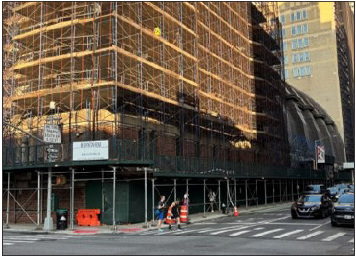
The outside of the Lexington Avenue Armory, which was built in the French "Beaux Arts" style between 1904 and 1906, is also being renovated as part of a $132.8 million contract.
