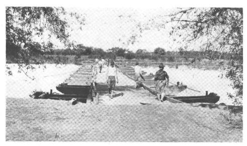
Heavy pontoon bridge erected by the 22d N. Y. Engineers west of Mission, Texas
