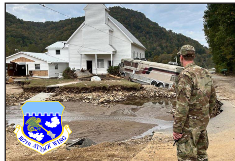
An Airmen assigned to the New York Air National Guard's 107th Fatality Search and Recovery Team surveys damage in the vicinity of Burnsville, N.C., while assisting the North Carolina National Guard in responding to Hurricane Helene. The 11 Airmen of the 107th Attack Wing's FSRT are trained to find and retrieve the bodies of those killed in disasters. Photo by Capt. Shawn Lavin, 107th Attack Wing.
